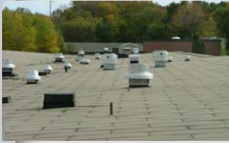
A view of the roof over the elementary wing.
